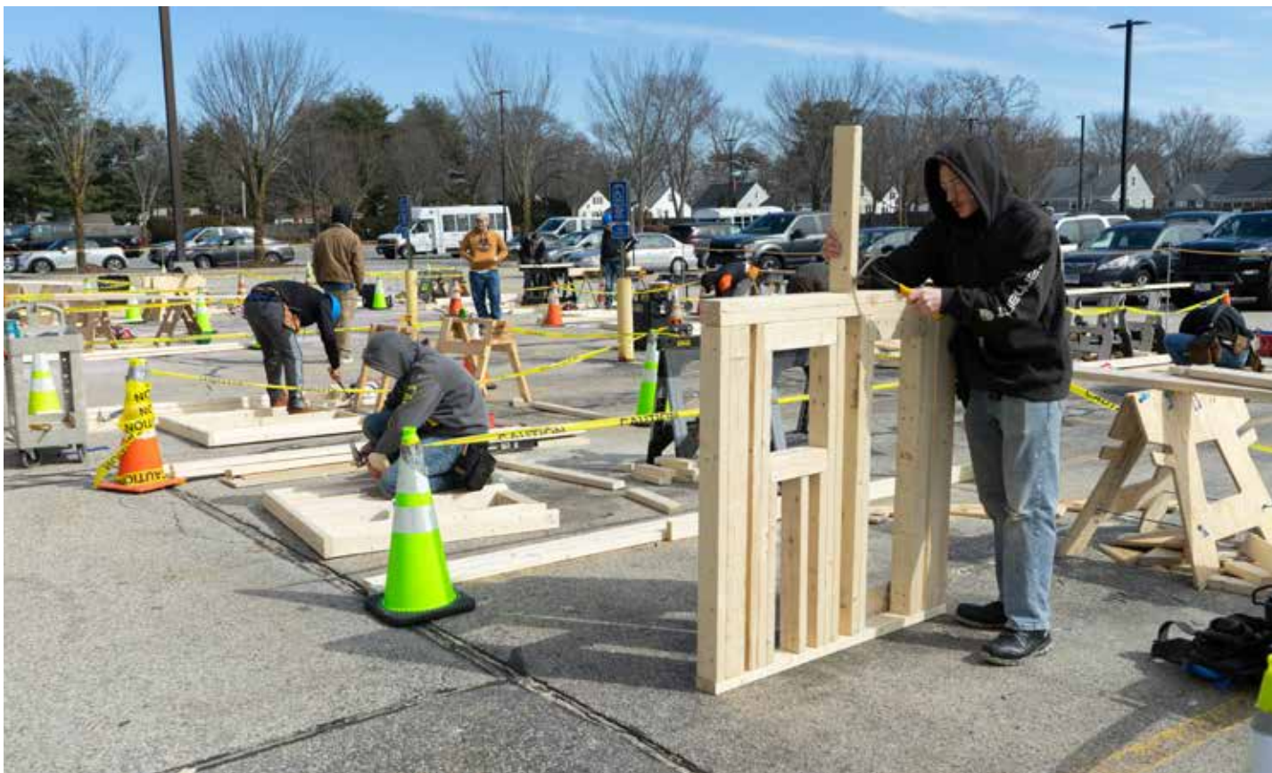
Students are framing a wall with door and window rough openings, as well as laying out a gable roof, based on the blueprint provided for the SkillsUSA carpentry competition which was held at NEIT's Post Road campus.
